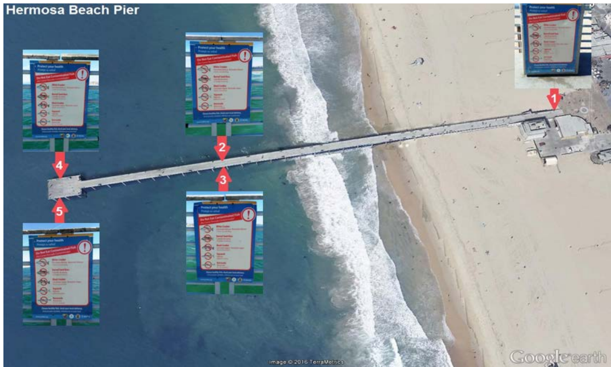
Hermosa Beach Pier: five signs total. One sign missing (#1) and needs replacement.
