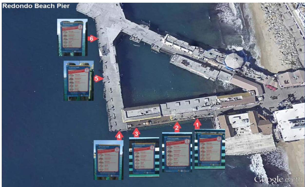
Redondo Beach Pier: Six total signs. One sign cracked (#6) and needs replacement.
