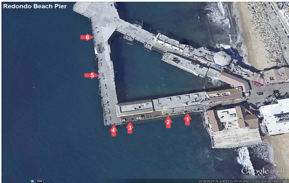
Redondo Beach Pier: Six signs total. No signs need replacement.
