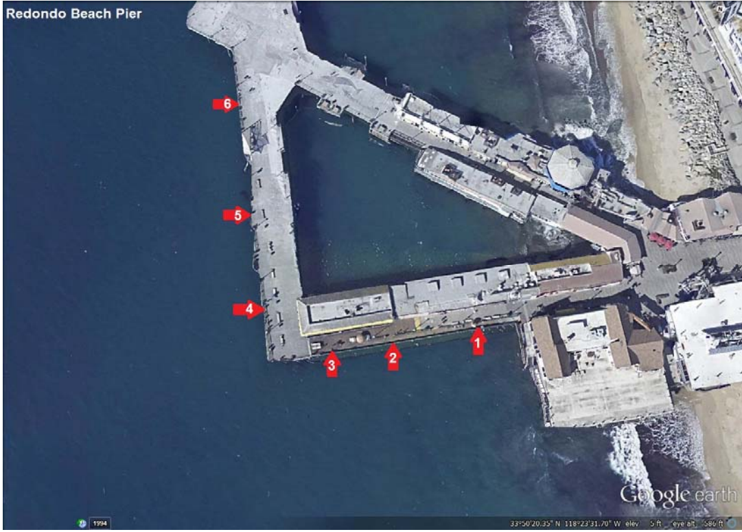
Redondo Beach Pier: Six total signs. No signs need replacement.
