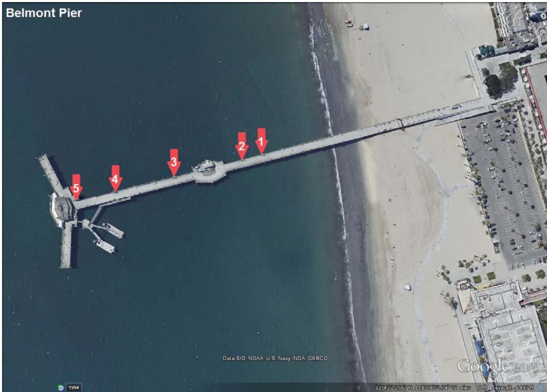
Belmont Pier: Five signs total. No signs need replacement.
