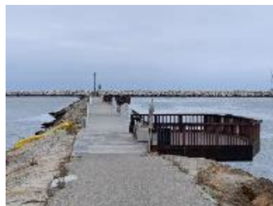
Piers at Ballona Creek
