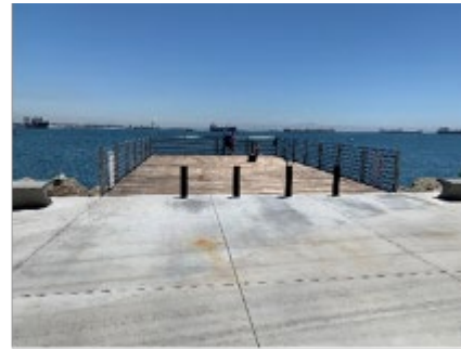
Pier south of Sign #1
