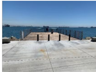
Pier south of Sign #1
